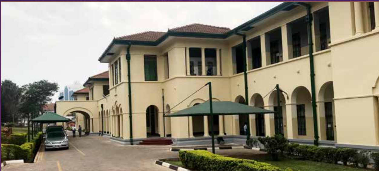
Refurbished: The new-look of Judiciary Head Office which was freshly renovated. The Northern and Southern parking drives were paved and marked, and the High Court Grounds were also greened, for the first time since 2008.
